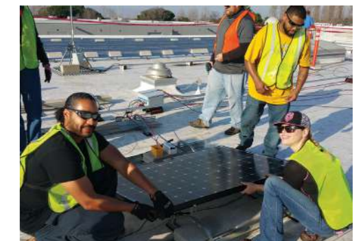
Teamwork to take this roof solar
